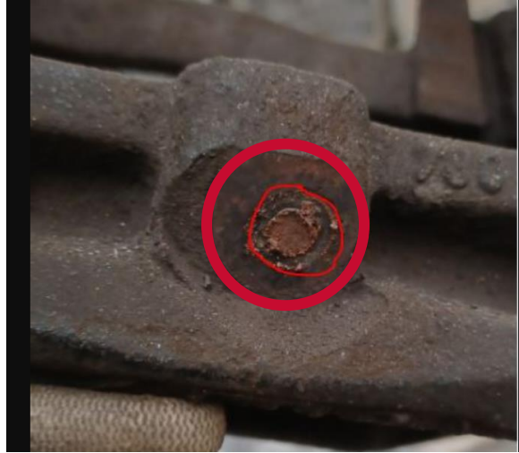
Cut screw (corrosion)
