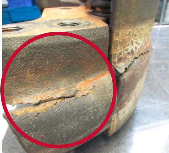
Cracked frame or carrier
